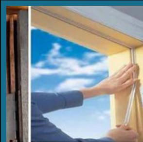
DOORS AND WINDOW INSTALLATION
